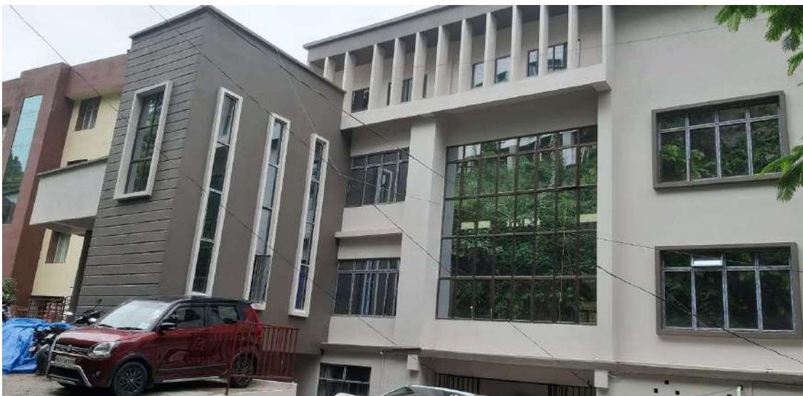
New Building, Directorate of Nursing, MINECO Khatla.
