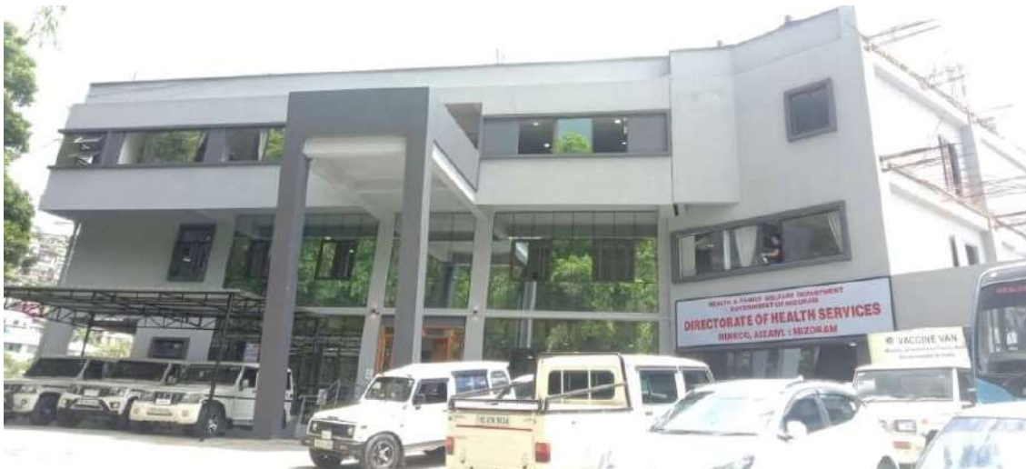
DHS New Building, MINECO, Khatla
