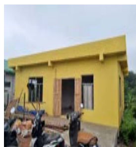
UHWC at Pukpui Lunglei
